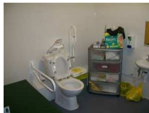
Nursery Accessible WC
